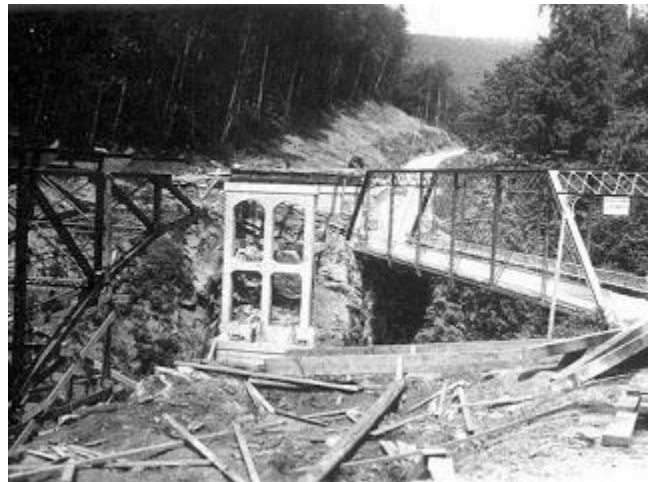
Building the third bridge next to the second bridge.
