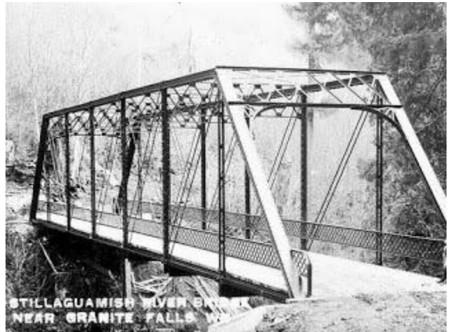
The 7-ton weight limit bridge
