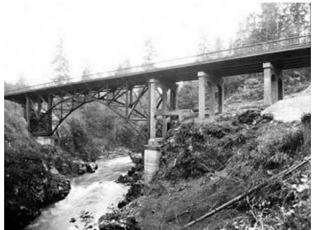
The third (and current) bridge.
