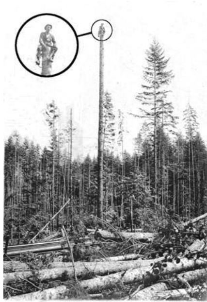
This fellow has finished preparing a tree to be rigged as a spar tree.
