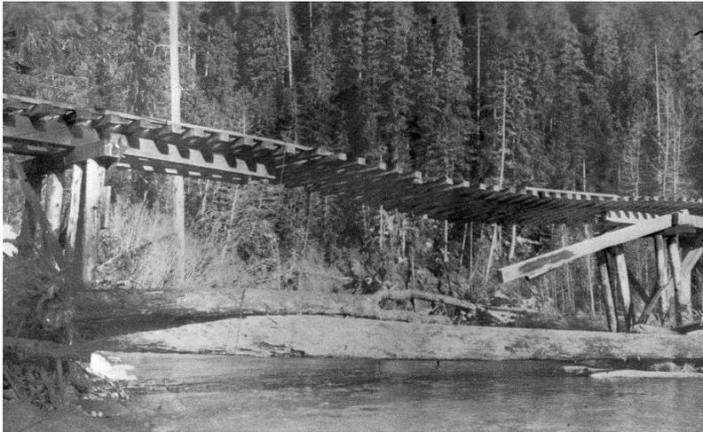
**When a raging river washed out the trestle supports, it was not uncommon for the rails and ties to remain (spiked together), simply swinging across the gap.**
