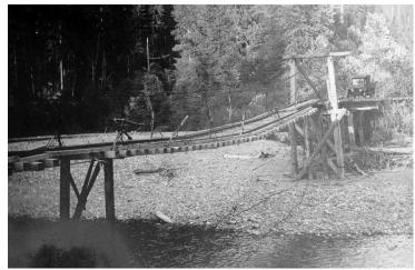
Ingenuity was important in bridge design, as well. Near the large Big Four Inn hotel was a bridge that allowed visitors to walk to the ice caves and beyond. A suspension bridge by design (unlike Red Bridge), it included hinges on its deck, to allow the deck
